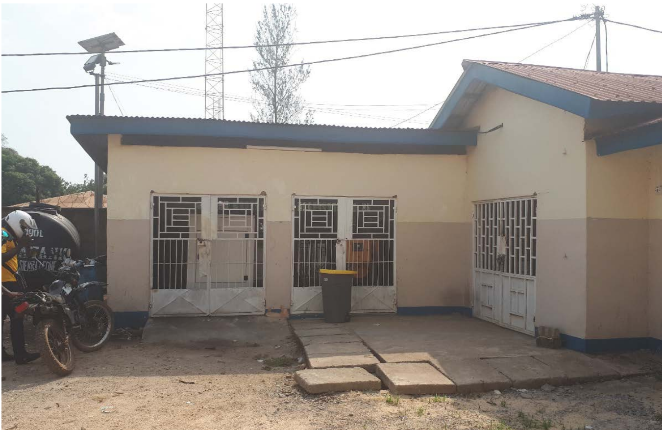
Image 9: Four generators supplying Koidu government hospital with 24 hour electricity (requiring 10.000-13.000 litres of fuel per month, estimated to costs ~7500 GBP). Photo by Eva Vernooij, March 2019.
